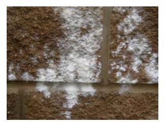
An example of efflorescence caused by calcium chloride in concrete.
